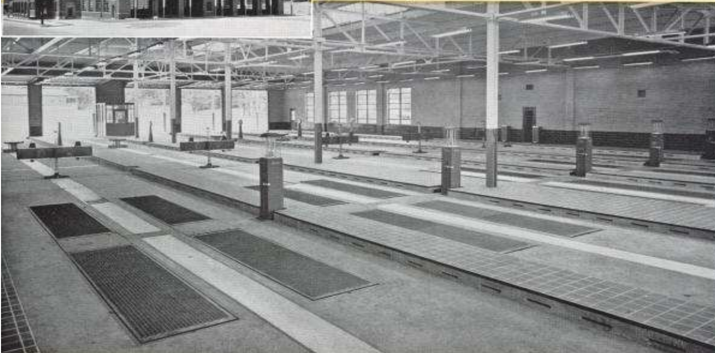
Illustration at left shows outside of new City of Memphis Official Inspection Station located at 150 High Street —Large picture shows 5 Weaver Safety Lanes in the Memphis Station.
